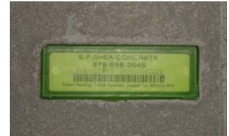
RFID tags can be embedded in a concrete structure
